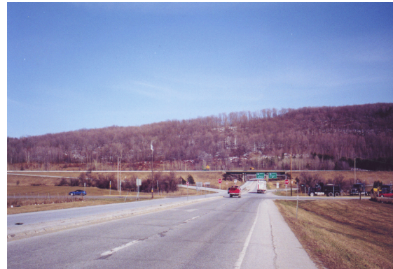
FIGURE 2 - Eastbound View of Intersection
